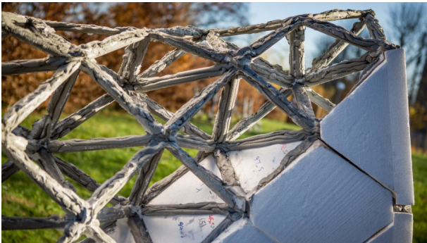
(c) The completed truss, after removal of some EPS blocks (photo: Stefano Borghi).
